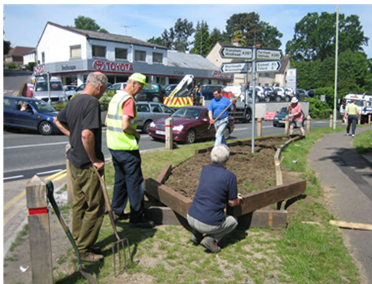
Building the first flower bed at The Bourne Crossroads, 2005
