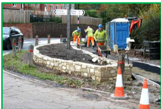
Construction work in progress
